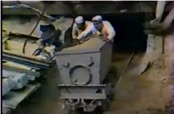
Miners removing earth from the tunnel. They dug directly under the core as it melted down.
