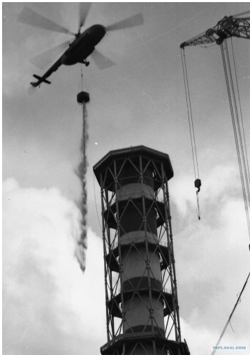
A helicopter drops a mixture of sand and boron onto the burning reactor
