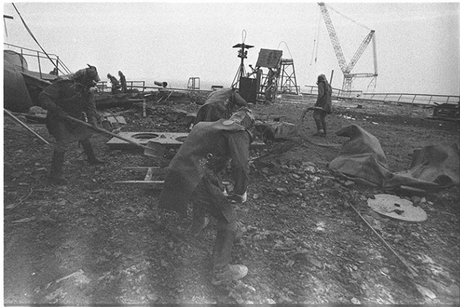
The "biorobots" of Chernobyl clean deadly debris from the reactor roof. Even with full protective gear, each would receive a lifetime dose of radiation in 90 seconds.
