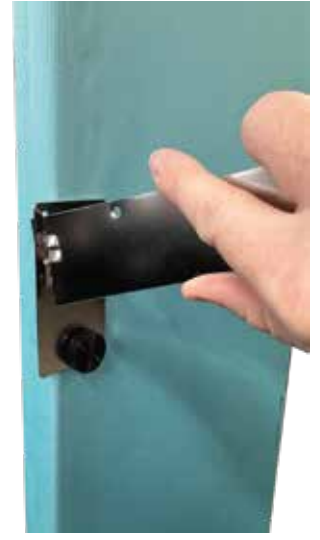
Bracket connecting to plate. Repeat for each shelf location
