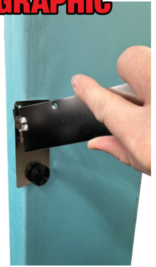
Bracket connecting to plate. Repeat for each shelf location
